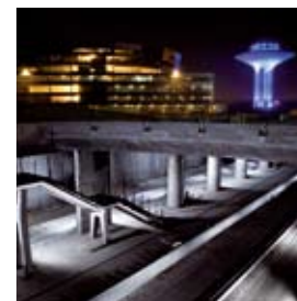
NVS AB is providing many of the installations for Malmö's Citytunnel Project. The project includes heating, sanitary and fire extinguishing systems at the stations and in the tunnels.
