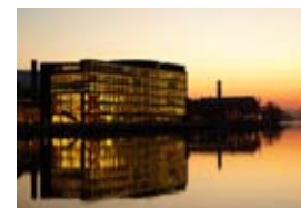
Drammen's Kunnskapsparken has premises for 900 university students. Besides heating, cooling, sprinkler and sanitary installations, NVS AB also provided a snow melting facility here.
