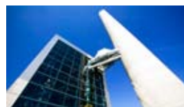
At the combined heat and power plant in Torsvik just outside Jönköping, NVS AB installed heating, sanitary, control, ventilation and flue gas cleaning systems.
