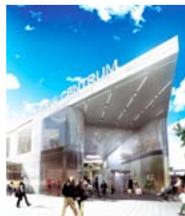
Sollentuna's main shopping mall is undergoing major restoration and expansion. This includes heating, cooling and sanitary installations by NVS AB.
